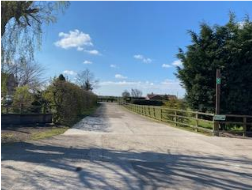
Photo 1 view to the exit and main road. There is a gate at the end and a small area for cars to pull in
