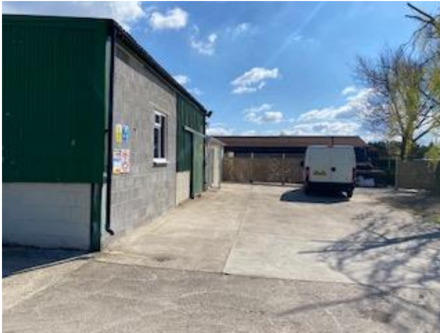
Photo 7 view outside showing the start of the potential outdoor seating area
